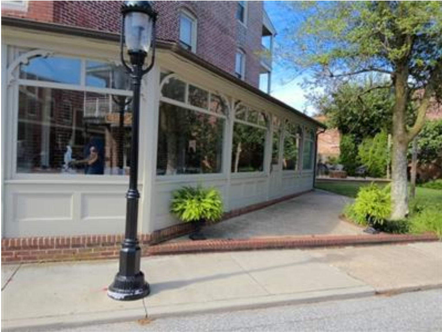
Looking from the corner of South Main Street and Broad Street
