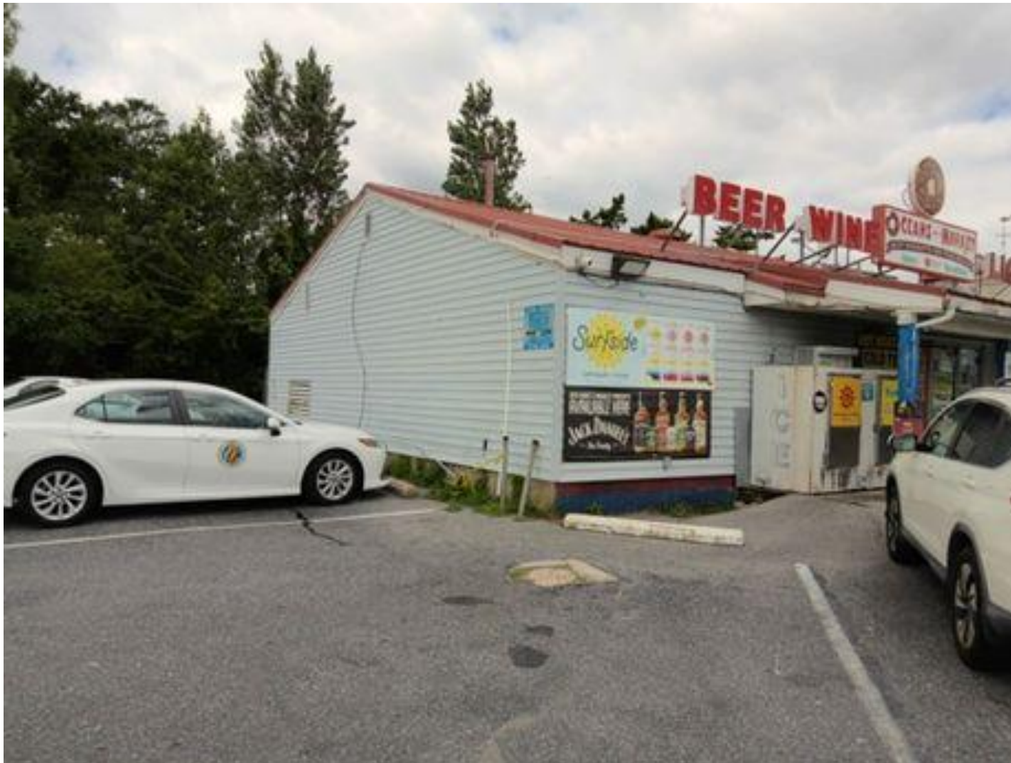
Looking outside at the south side of the building
