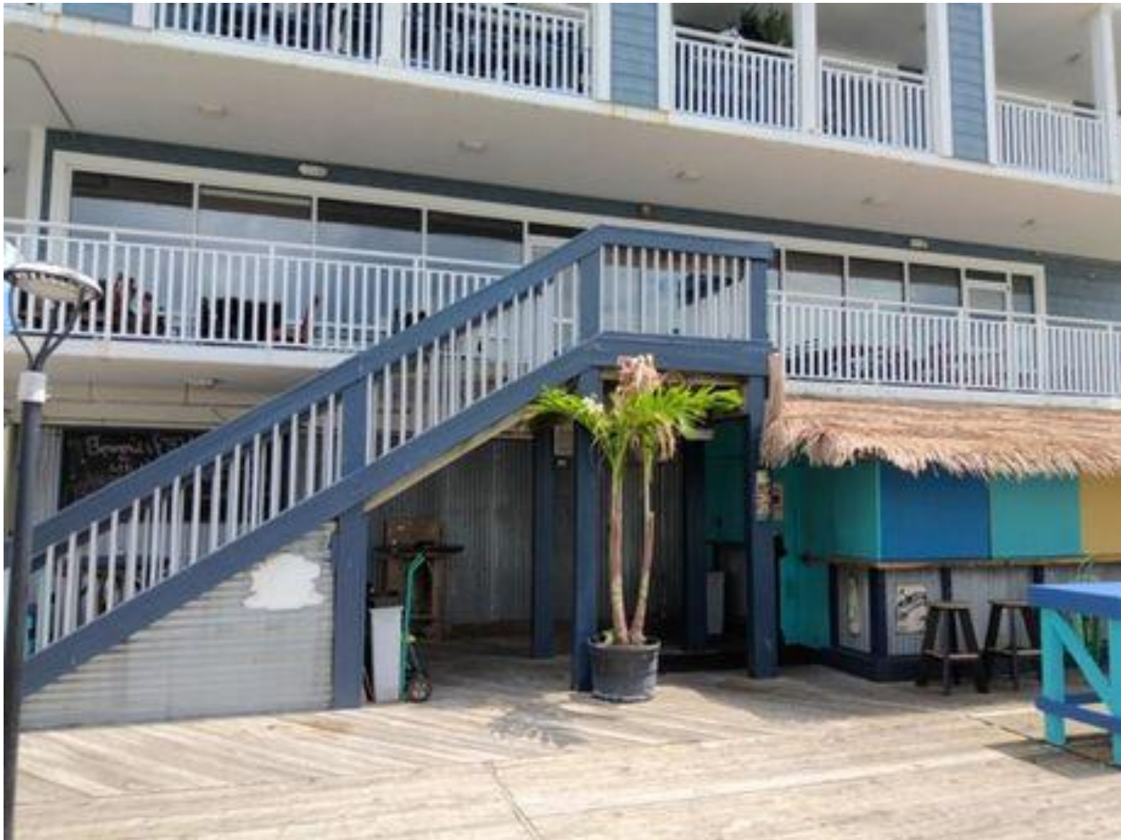
Looking from first floor deck to second floor patio
