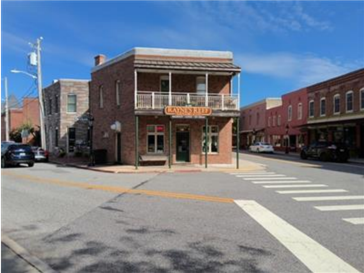
Looking from Broad Street side of the Hotel
