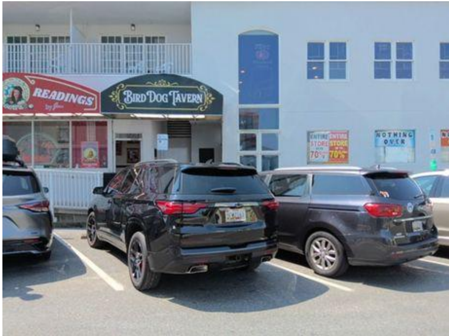
Front entrance from 9 th street
