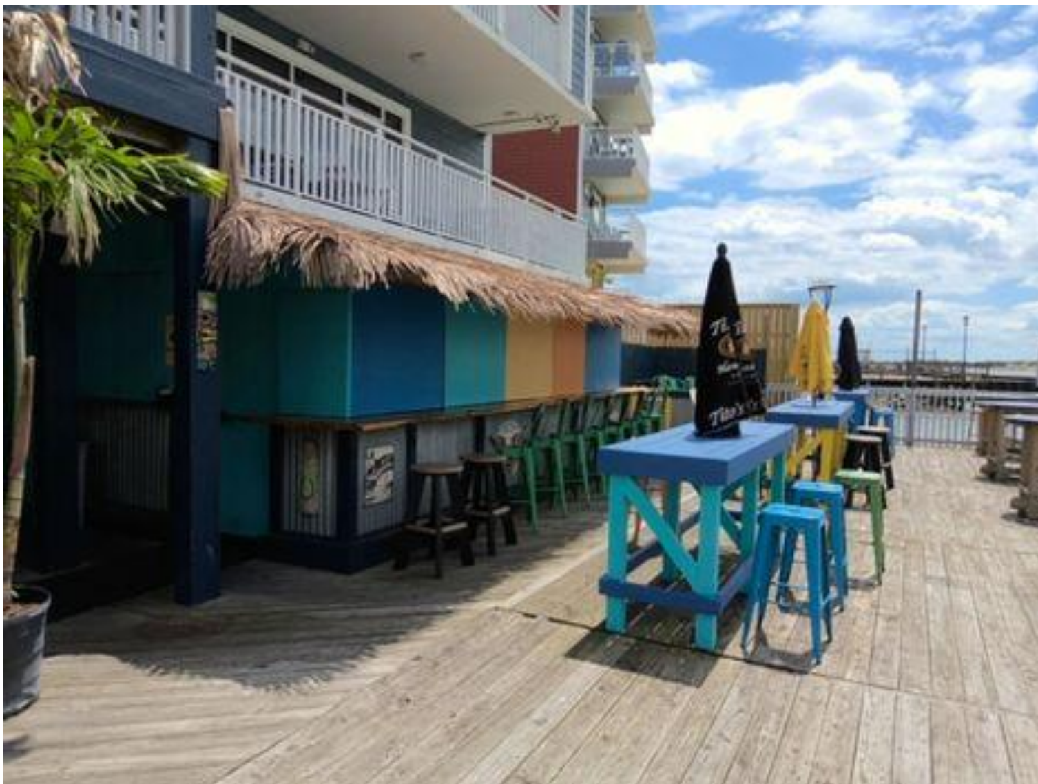
Looking at the first-floor deck outside bar
