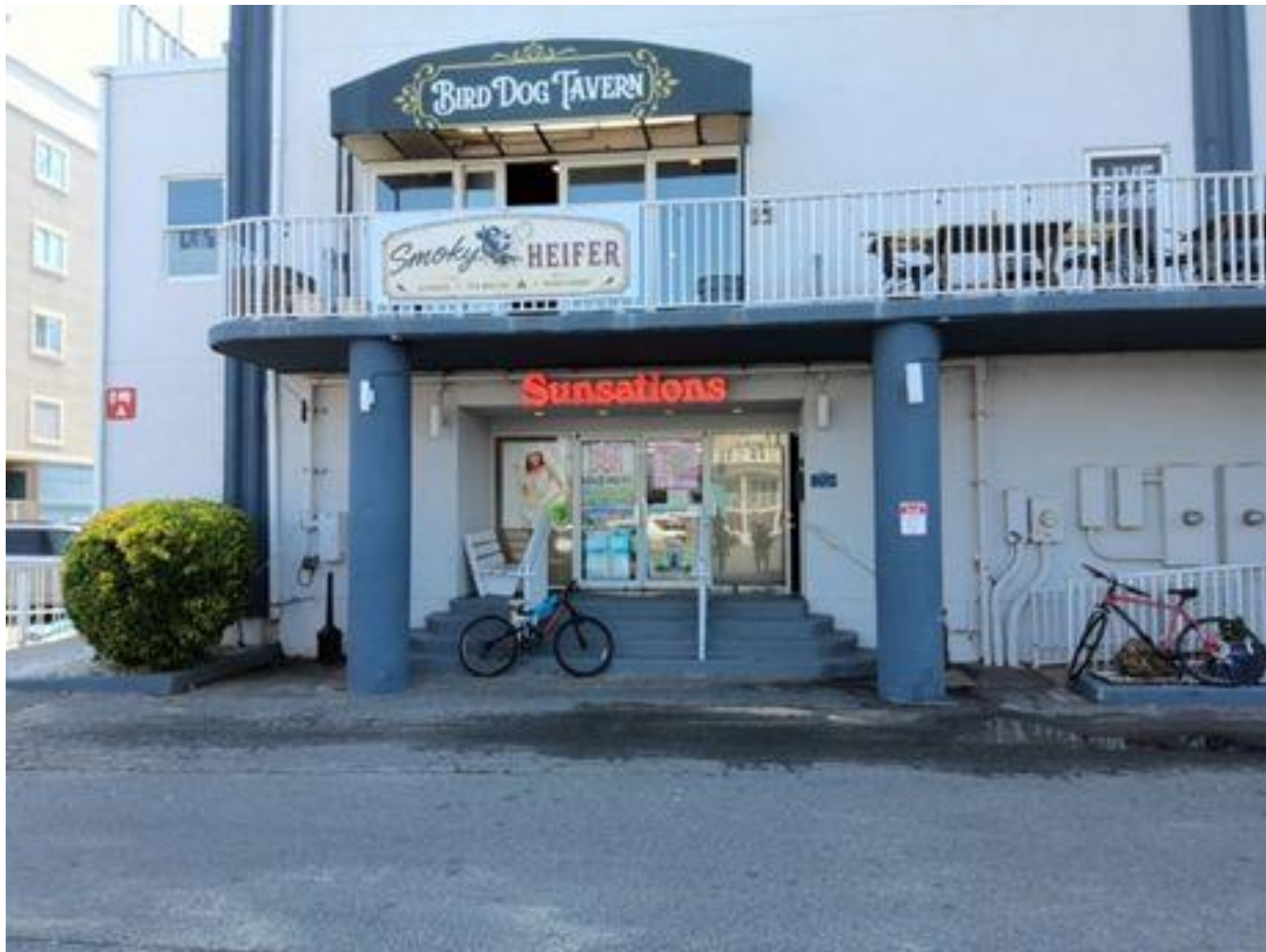
Back entrance/ side door to building
