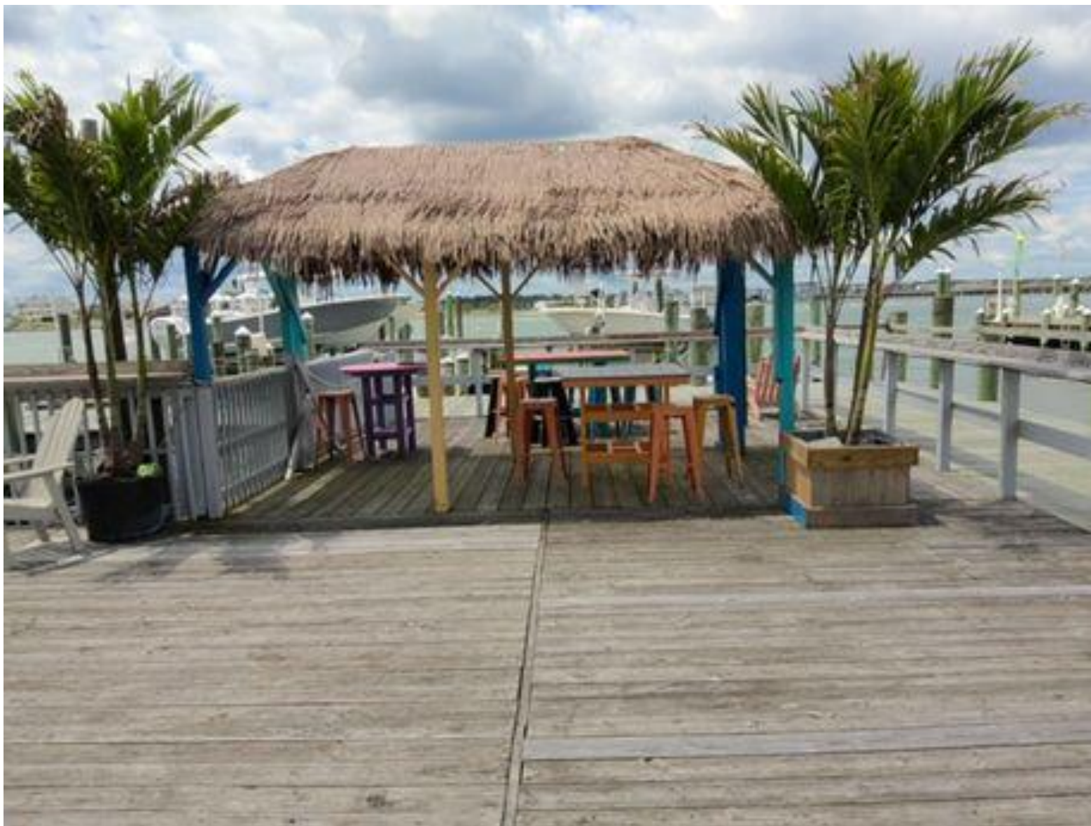
Looking at first floor deck with covered area
