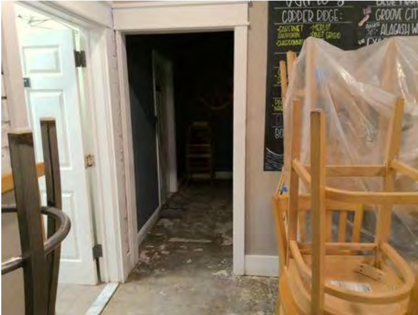
Right side of Restaurant looking at the back. Restrooms
